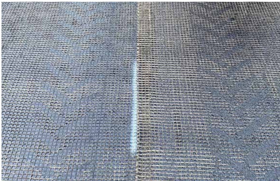
Overlap sidevejs med markeringsmærke ved 10 cm overlap
