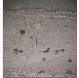
The highway inspection revealed that there was severe cracking on the road surface.
