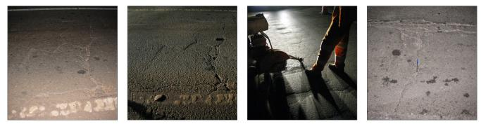
The highway inspection revealed that there was severe cracking on the road surface.
