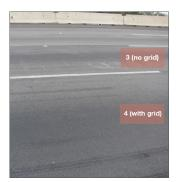
Whilst lane 4 remained in good condition, lane 3 was yet again showing signs of heavy damage and in need of repaving for a third time.
