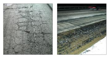
The road surface was milled and the S&P asphalt reinforcement grids were laid onto bitumen tack coat.
