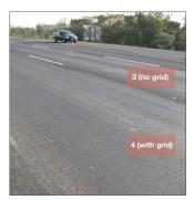
Lane 4 repaved with S&P asphalt reinforcement grids in April 2011, Lane 3 repaved without grids in May 2011.
