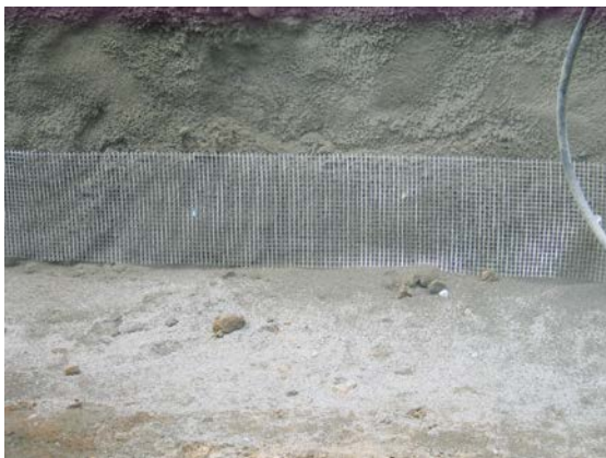
Figures 15 / 16: Local strengthening at anchor heads
