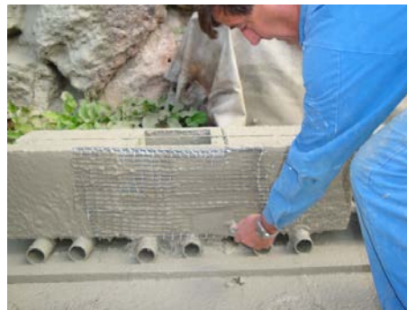
Figure 4: Application of spray mortar and S&P ARMO-mesh L500
