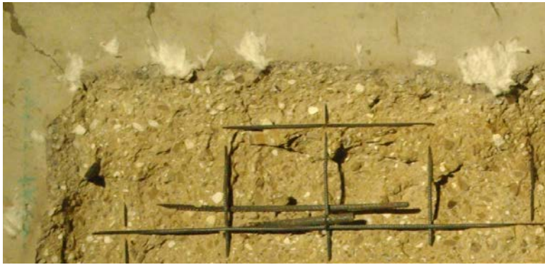
Figure 32: Spalling of a structural concrete surface
