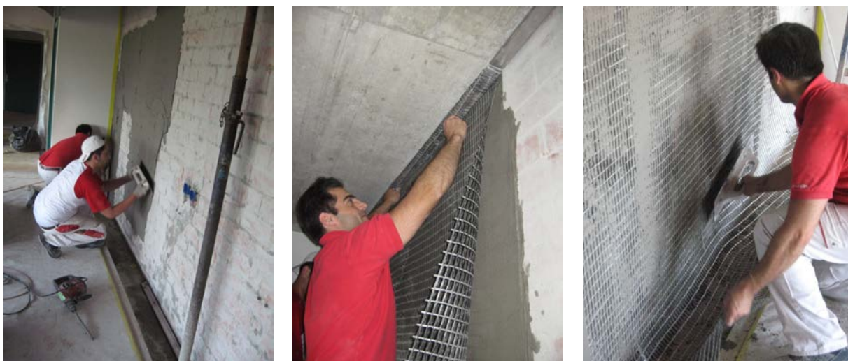
Figures 26 / 27 / 28: seismic strengthening and anchorage of a masonry wall using S&P ARMO-mesh
