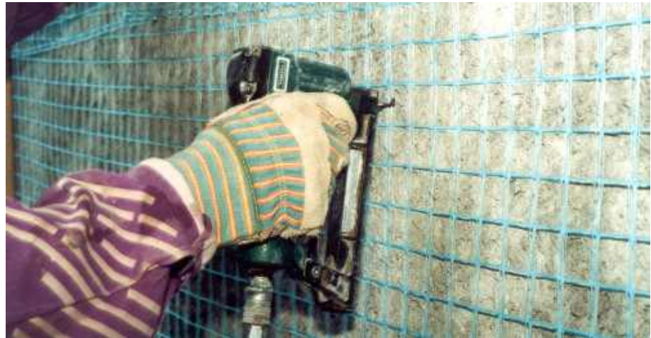
Figure 14: Fixing of S&P mesh using clamps
